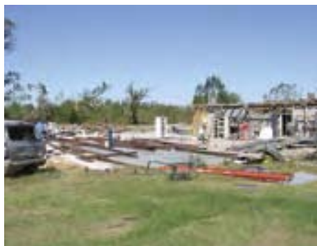
Garage flattened by the power of the storm
