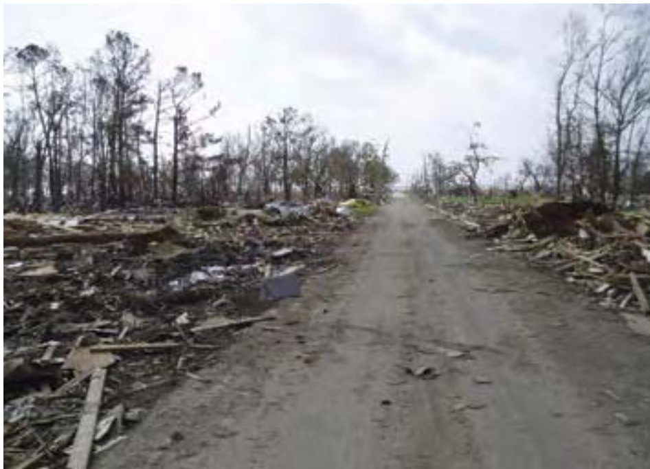
View of the surge zone near the Gulf coastline shows very little left standing
