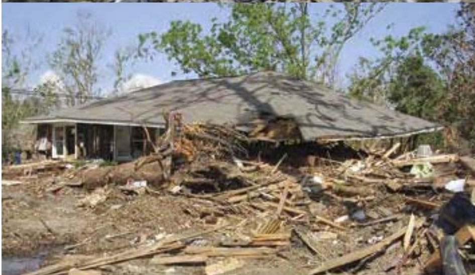
Examples of the total destruction in Long Beach, Mississippi
