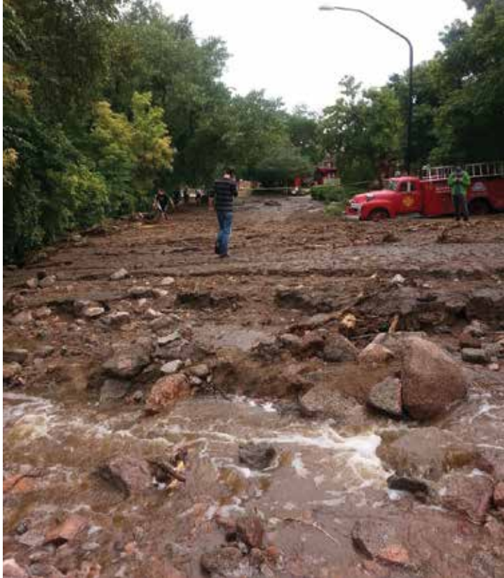
Arapahoe at 1st street on Sept.13, 2013. Flood brought debris onto the road and caused serious damage.
